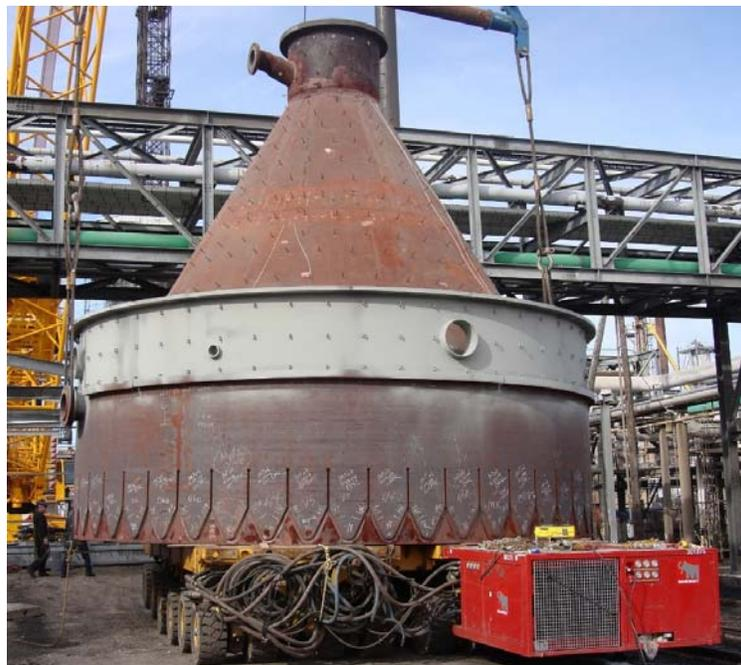
Fig. 4 – T-Rex Skirt for Frontier El Dorado Coker Project
